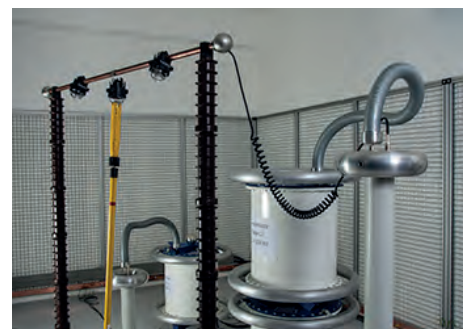
High voltage laboratory
